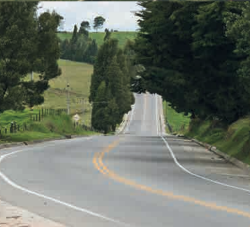
Technical supervision for the improvement of Hatillo – Caucaasia roadway Colombia
