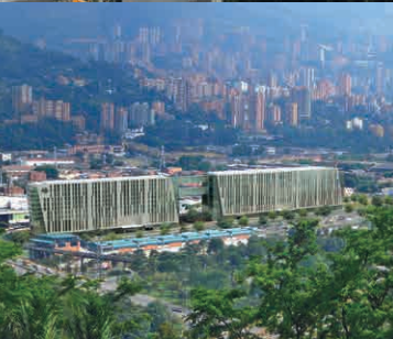
Building Automation System and electrical system design of BANCOLOMBIA S.A financial organization Colombia
