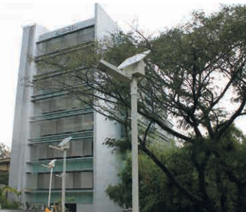
Design and equipment specifications for the electric, sound and telecommunications systems of the ISAGEN S.A Energy generation and commercialization Company Colombia
