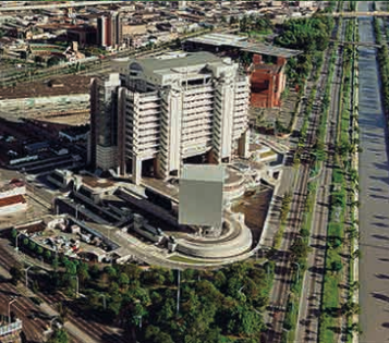
Building Automation System, electrical system design and construction engineering of EPM S.A E.S.P Public utility Company Colombia
