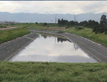
Detailed designs for the sanitary and storm sewer of El Tintal basin Colombia
