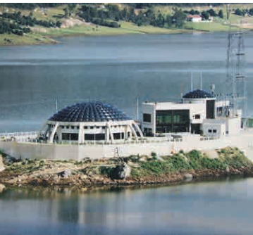
Supervision during the construction of the pumping station and ancillary works for the San Rafael Reservoir Colombia
